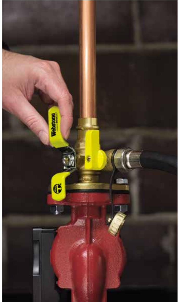
Use a uni-flange ball valve to isolate pumps for service.
