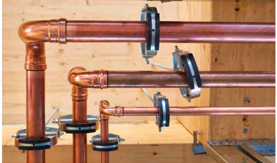
Viega's two new buildings use ProPress fittings behind the walls to provide potable water because, as Braconier President Tom Stone said, soldered joints might leak, but ProPress joints do not.
