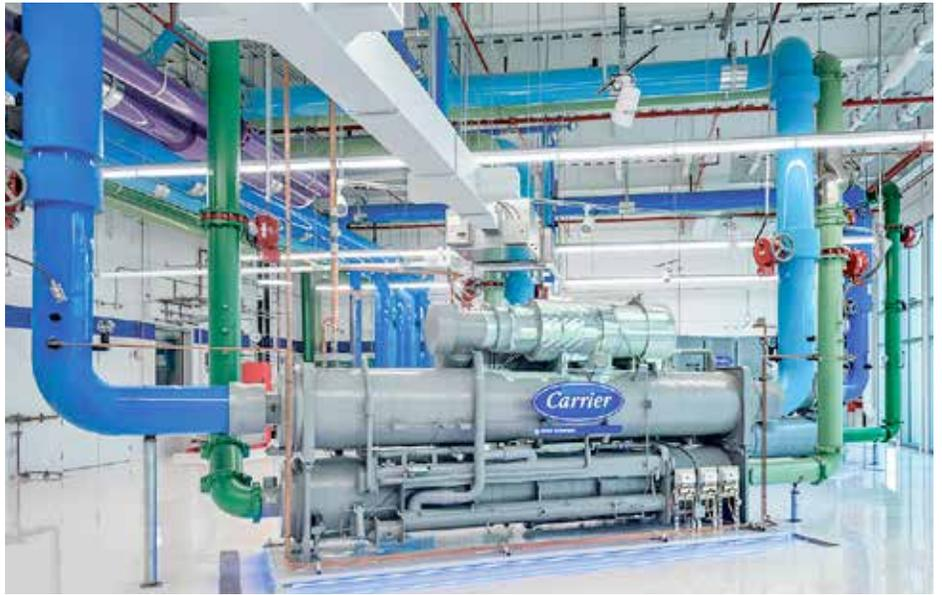
**Right:** To shave time off the installation timetable, Hill York prefabricated offsite many of the piping components that typically would have been done onsite for Carrier’s new headquarters.
