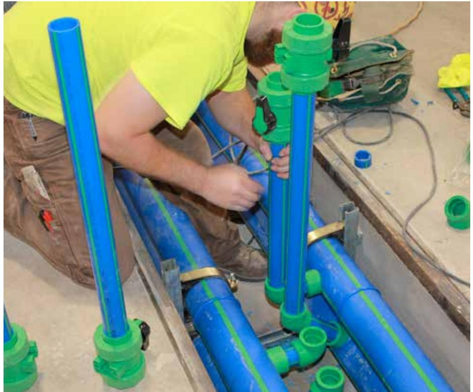
Warner Mechanical found that Aquatherm polypropylene pipe was ideal for the new IVP Plastics facility, and it is easier and faster to install than traditional welded pipe, saving the contractor time and money.
