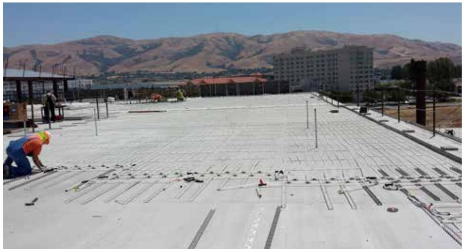
ACCO crews installed 138,000' of tubing with Uponor's Radiant Rollout Mats in five months at Delta Electronics (Americas) Fremont, CA, headquarters—much faster than the time required for conventional PEX rails or tie-down methods.
