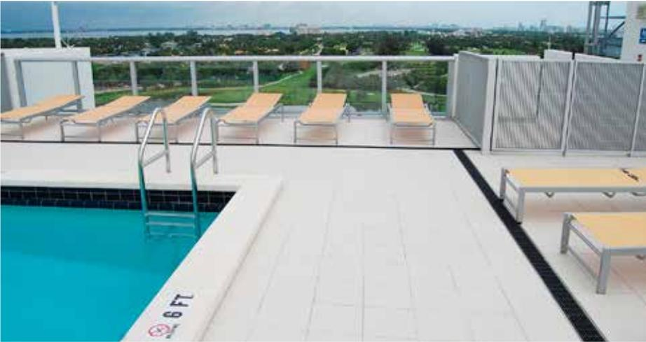
Stainless steel was specified for this pool because it is long-lasting, does not harbor bacteria, and can stand up to pool chemicals. A ductile iron grate was selected to prevent bathers from slipping.
