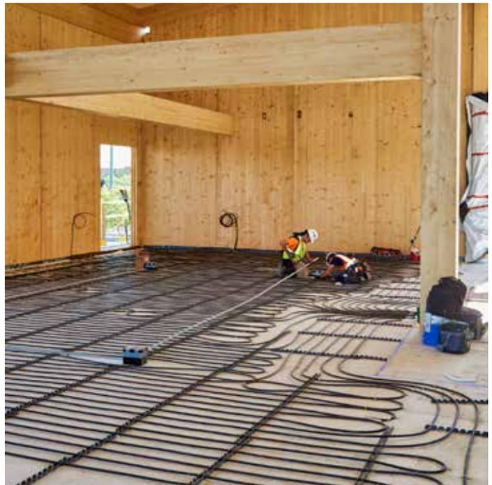
The radiant system in the seminar center—which contains more than 36,000 linear feet of tubing—was the largest Braconier had ever installed. The bare concrete floors stay comfortable year-round with the radiant products.
